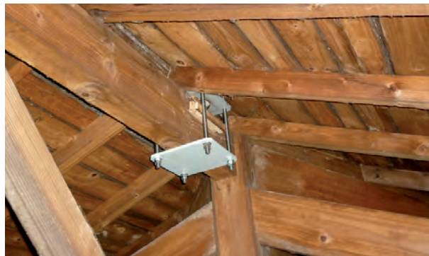
Ancrages potelet (photo Somain)
